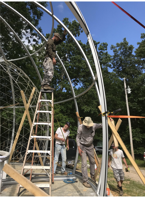
The 28' polycarbonate dome – "Wholeover" - is assembled.
