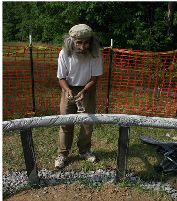
Francesco Casini built the 14 posts and concrete ring.
