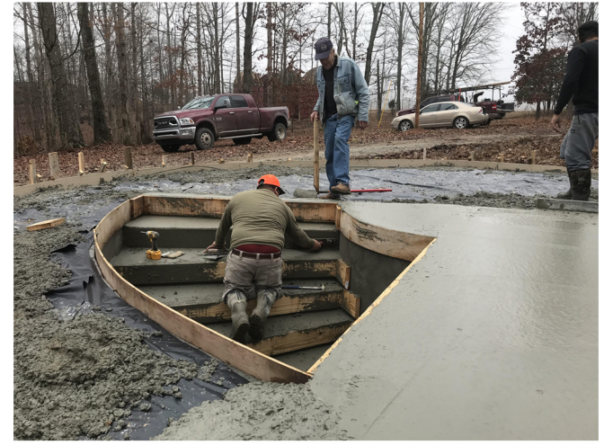
JaySun designed the perfect stairwell, keeping the dome's curve.
