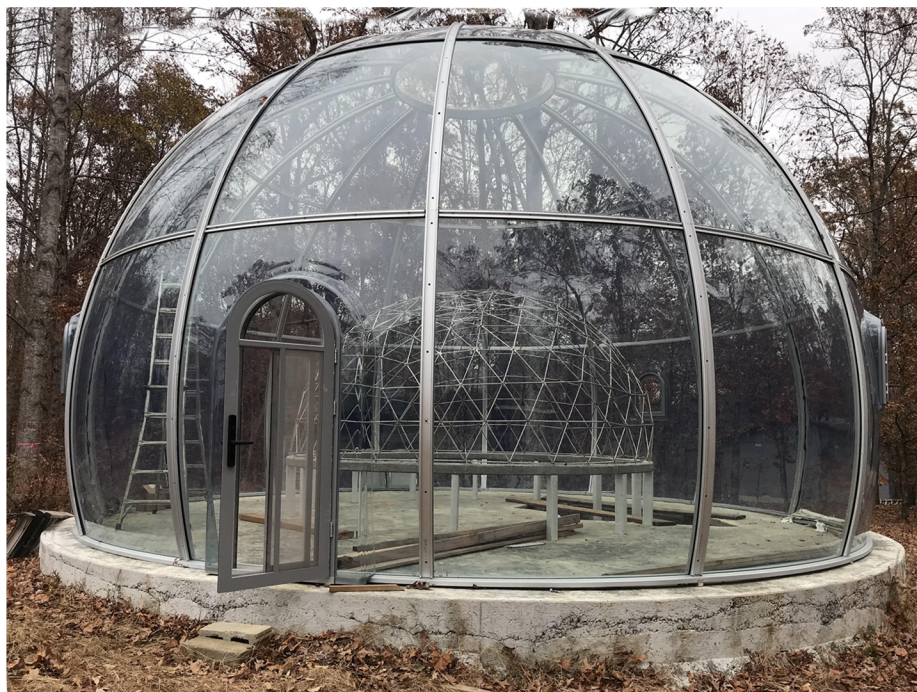
"Wholeover" is complete - a door that locks and 4 windows. The geodesic dome inside waits for Wholeo's panels.
