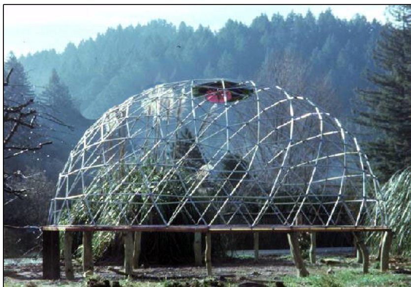
Wholeo with half the panels attached
