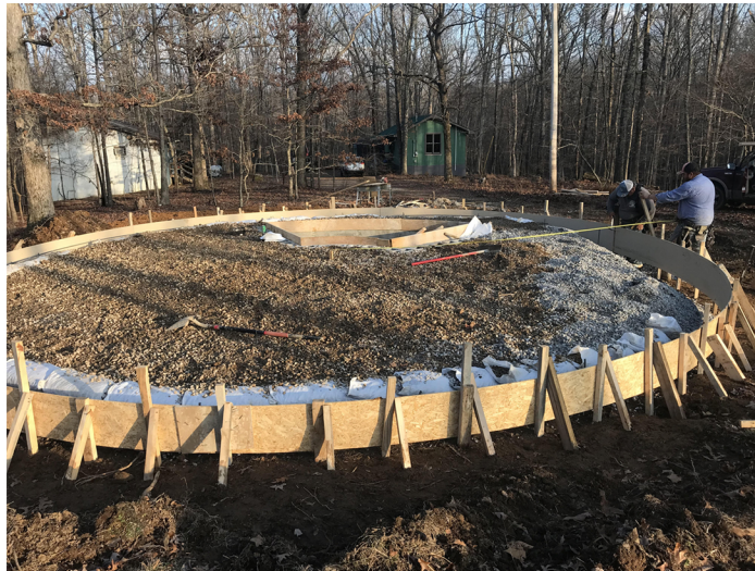
A new site was found, and the foundation is prepared.
